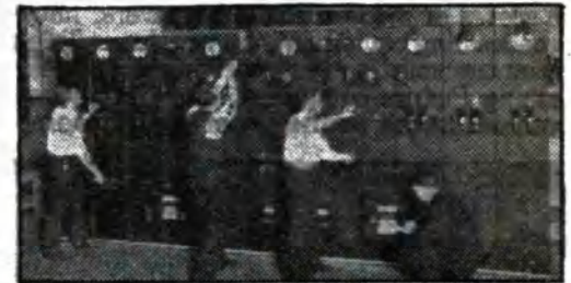
Students learning switchboard work by actual practice
